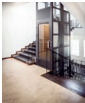
ELEVATOR INSTALLED INSIDE THE STAIRWELL
